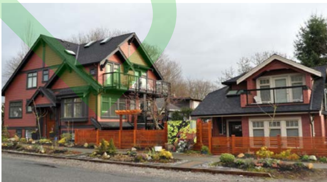
Figure 7: Example of a garden suite with an architectural style that complements the primary dwelling (photo: District of North Vancouver )
