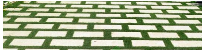
Figure 21: Example of permeable interlocking pavers (Photo: http://www.gtlandscaping.com )
