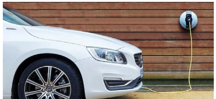
Figure 24: Example of a parking space with an energized outlet for an electric vehicle
